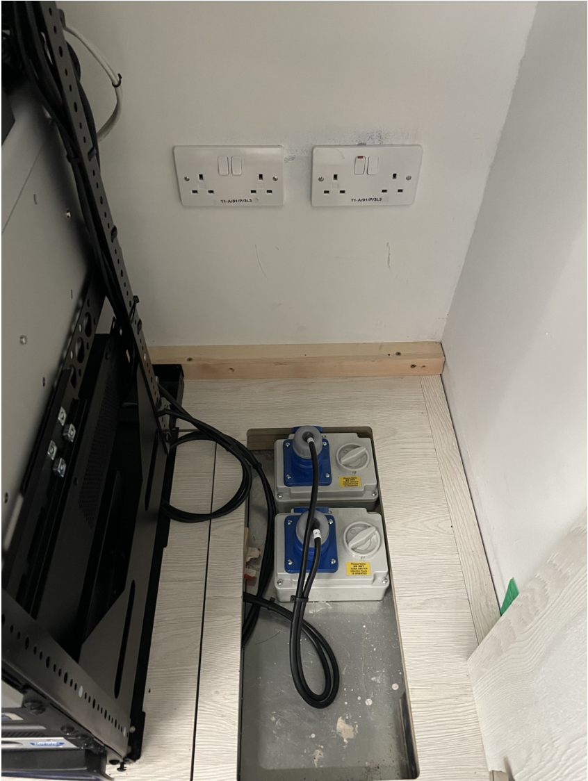
Rack 2 power on the right hand side of rack
