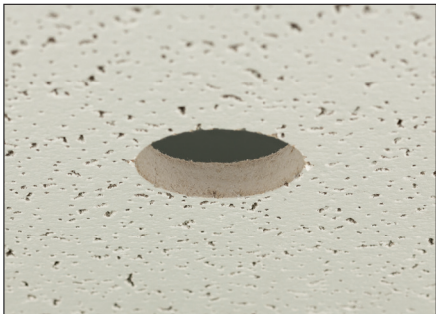
FIGURE 1 Determine the microphone placement, drill a 2 inch (51mm) hole in the ceiling tile or mounting surface.
